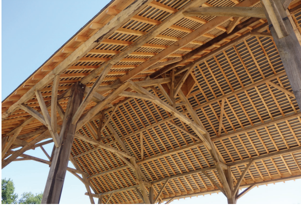
Communal hangar and atelier built at the zad. Photo K. Ross
